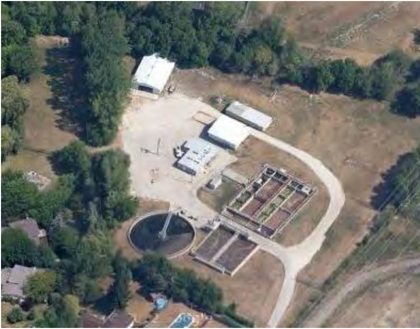
Derby Meadows Waste Water Treatment Plant facility. Source: Google.
