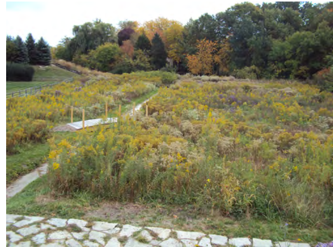
"Transformation Prairie" detention retrofit
