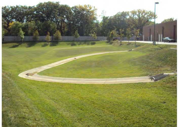
Typical dry bottom basin w/concrete channel behind Aldi, Lemont
