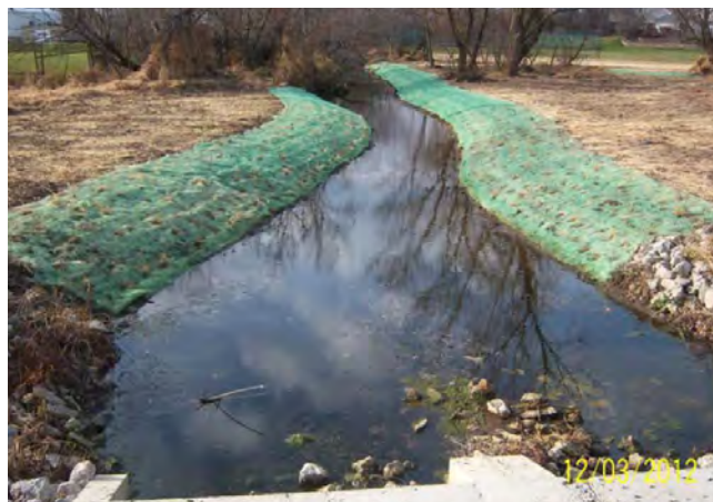
Streambank project completed by Homer Glen
