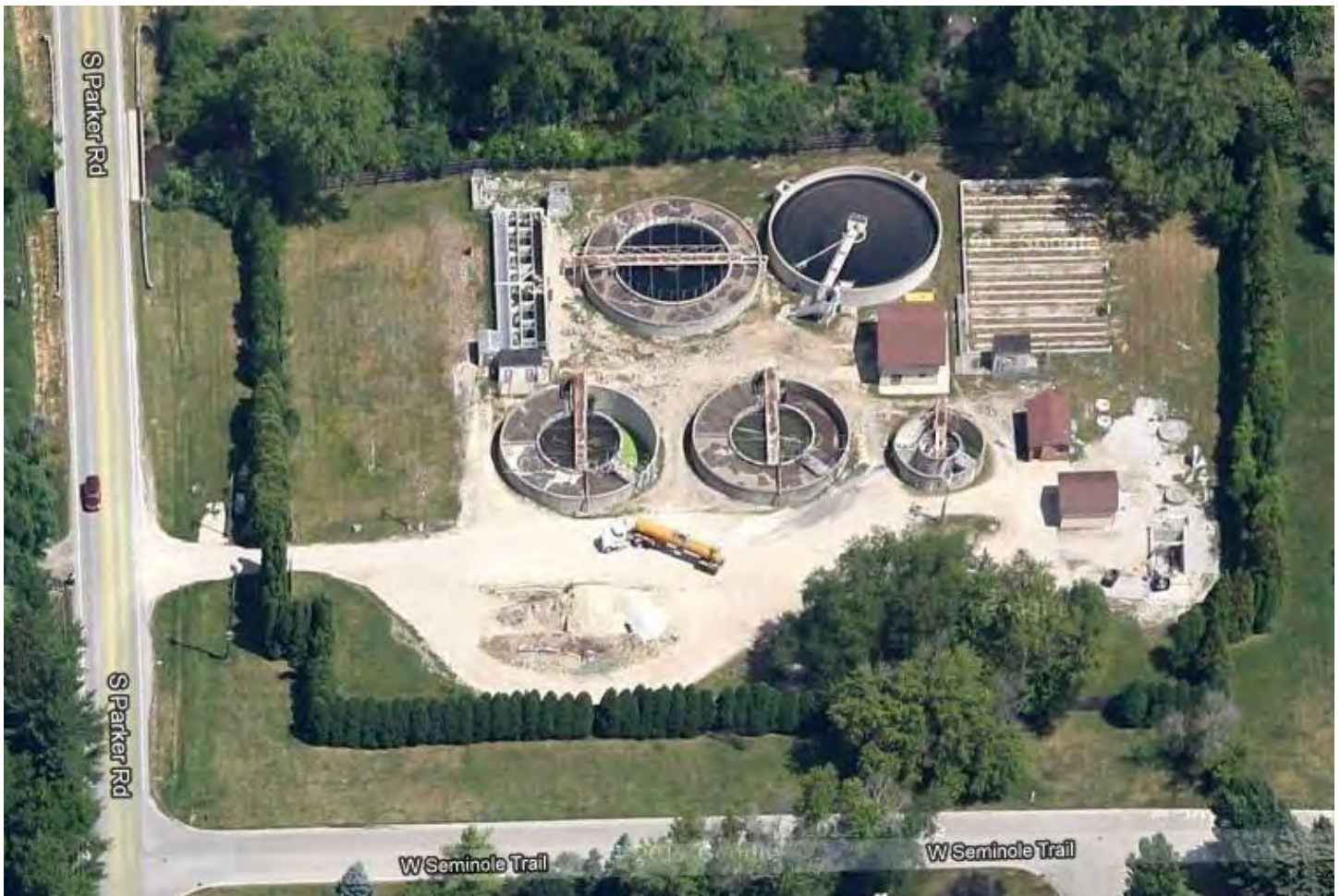
Chickasaw Hills Waste Water Treatment Plant facility east of Parker Road. Source: Google.
