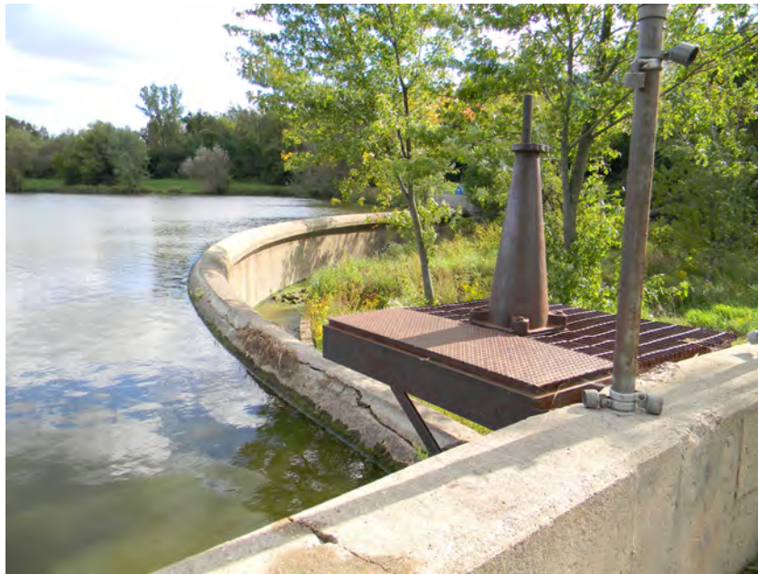
Dam at southwest end of Tampier Lake
